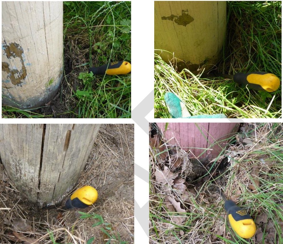
Inspecting for rot with a screwdriver
