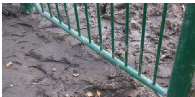
Mud at a gate shows effect of high wear and makes access difficult particularly for push/wheelchairs
