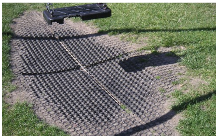
Grass unable to cope with scuffing even when reinforced with grass grid
