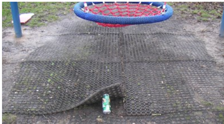
Both above photos demonstrate that, even with grass grid reinforcement the grass cannot cope with scuffing
