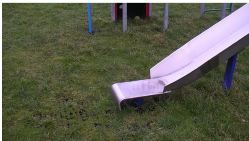
Patches only needed at areas of high wear (slide runout, fireman's pole etc)
