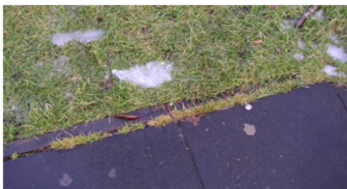
Grass encroaching naturally and filling the gaps as well as anchoring the edge
