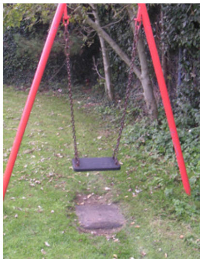
Rubber tile wear patch of slightly insufficient dimensions
